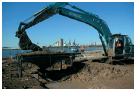
Work has started on the $110M remediation of the Mayfield site.
