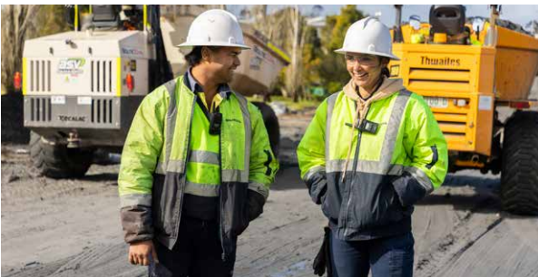
Encouraged Aboriginal participation in construction, women in construction and mental health awareness through the implementation of social media campaigns
